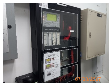
Fire Alarm Control Panel
