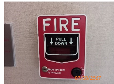
Fire Alarm Manual Station
