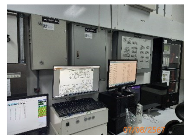
Graphic Annunciator Fire Alarm System
